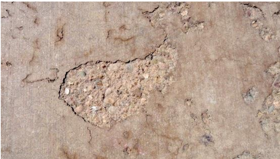
Small patches of flaking
